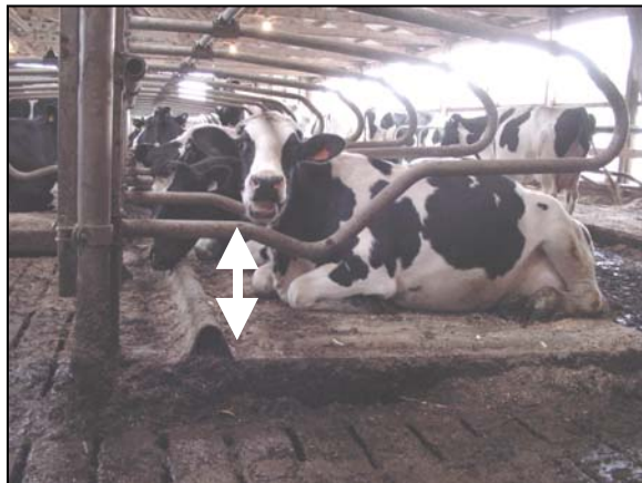
Figure 1 shows loops that are inappropriate for side-lunging stalls. The lower pipe of the loop is 18 inches above the bed. It is too high for normal lunging motions.
