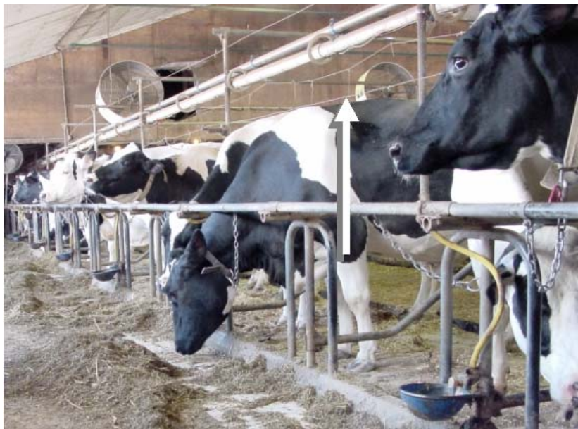
Figure 2. The photograph shows a single wire used as an electric cow trainer. This application has several flaws. The wire is mounted 56 inches forward of the gutter curb and low enough that it rests on the taller cows in the row. The wire is strung between posts at every 3 rd or 4 th cow. There is no provision for easy vertical adjustment for individual cows. The milk and vacuum lines are about 48 inches forward of the gutter curb - the preferred location for the electric trainer.
