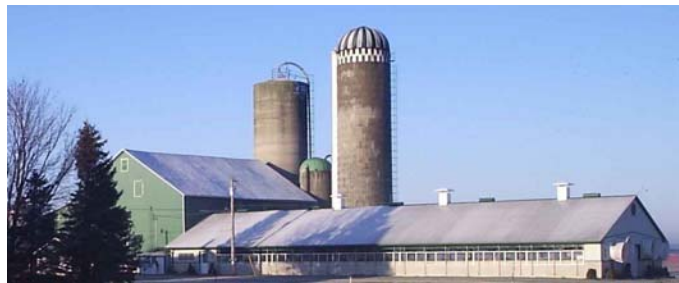
Photo 1. Tie-stall dairy barn with natural and tunnel ventilation
