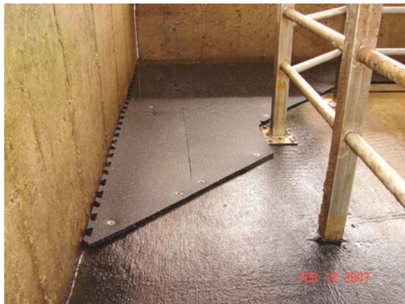
Figure 1. Return lane with rounded-off corner and rubber mats
