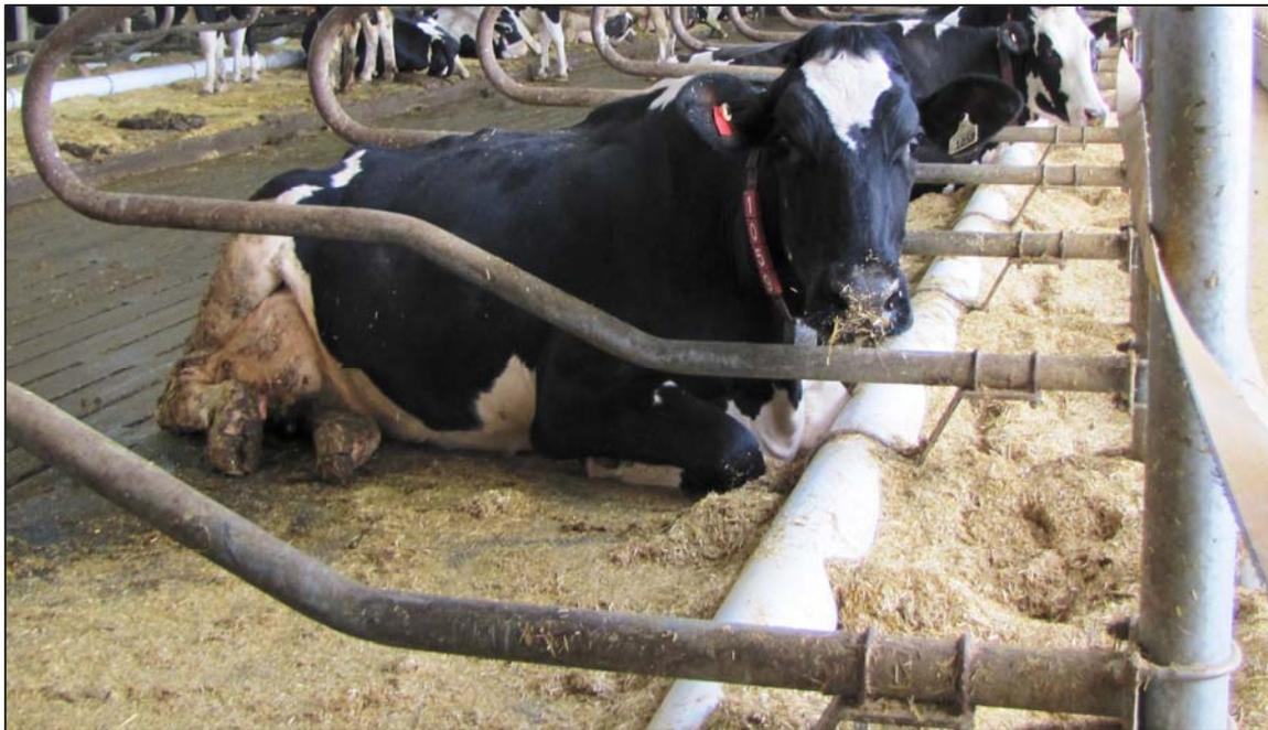
**Figure 2.** The 6-inch PVC sewer pipe shown in this photo is an innovation in a barn built in 2011. It attaches to the bottom pipe of a loop with metal bracket and provides a 3-inch space for trapping a front leg. It also is too high and too wide for a normal stride when rising and it is an impediment to the legs forward resting posture. It contributed directly or indirectly to injuries to cows in this barn.
