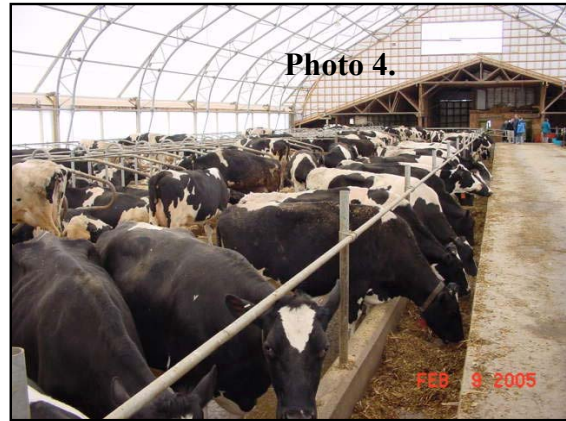
Photo 4. A new 4-row barn near Spencerville, Ontario has an elevated drive-through feed alley that provides a feed barrier.
