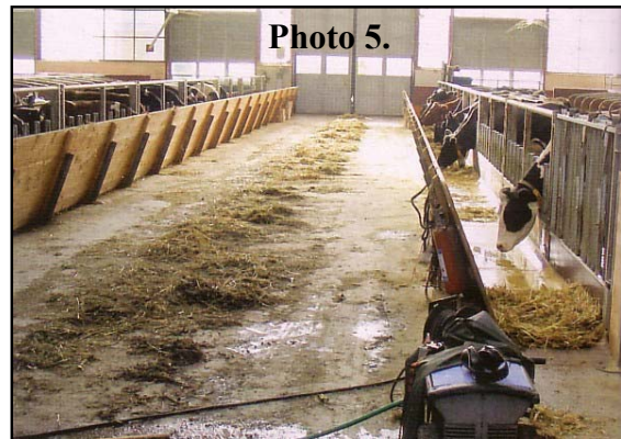
Photo 5. A sweep-in manger retrofitted with a wooden feed barrier.
