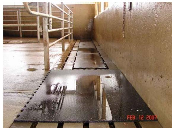
Figure 2. Slatted floor with rubber track to transfer alley
