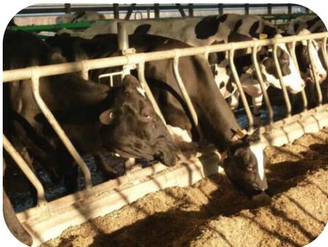
**Figure 1.** shows pre-manufactured slant-bar restraints installed on top of a 20-inch conventional curb at a feed bunk in a free-stall dairy barn. The mismatch of cow size (height) and slant-bar design is apparent because most cows contact the horizontal top pipe of the slant bar installation.
