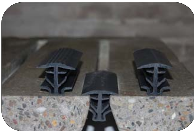
Figure 2. Slat gap filler inserted into cement slat (middle)
